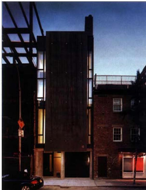
*The steel facade was installed in a single morning by Alcon Builders Group, which handled all construction. On the ground floor, Baird and the project architect Talia Braude put in a garage.*
